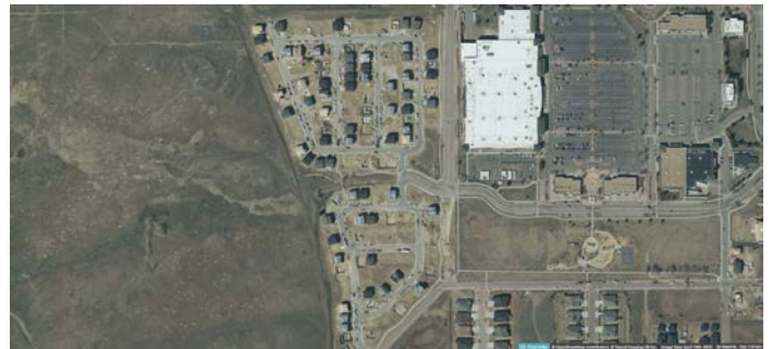
April 10, 2023. Imagery 16 months after the Marshall Fire shows the progress of rebuilding homes in the neighborhood.
